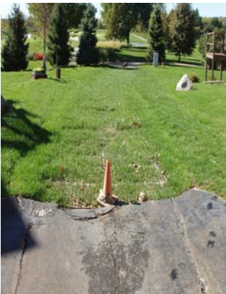
Vegetated drainage way able to exceed 15 lbs/ft2 shear stress.
